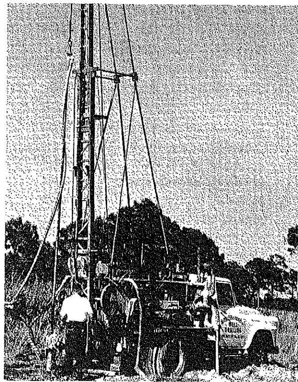
Fig. 5 Jet drilling operation.
