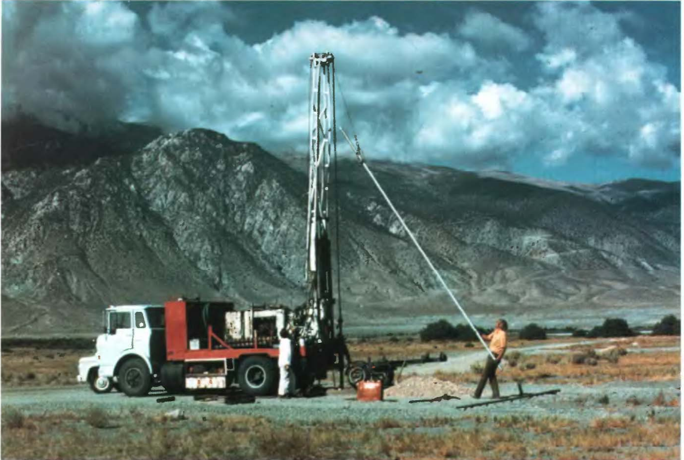
Exploratory well installation by the U.S. Geological Survey near Hawthorne, Nevada, September 1977. The study, at a military ammunition plant, indicated that liquid explosives wastes had percolated into the shallow basin-fill aquifer beneath disposal pits (Van Denburgh and Schaefer, 1986). (Photograph by A.S. Van Denburgh, U.S. Geological Survey.)
